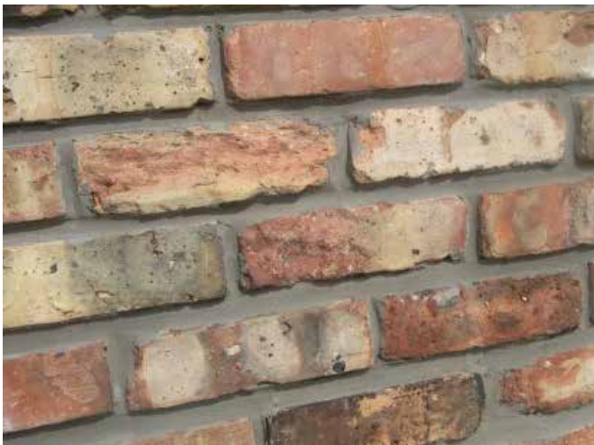
Figure 2.8 Re-used brick facade
